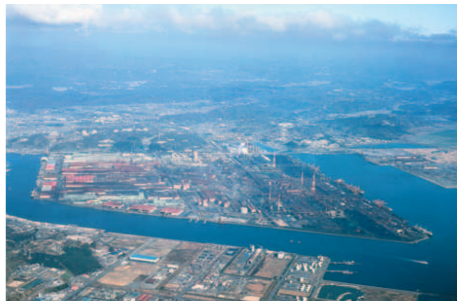
▲ West Japan works (Fukuyama)
